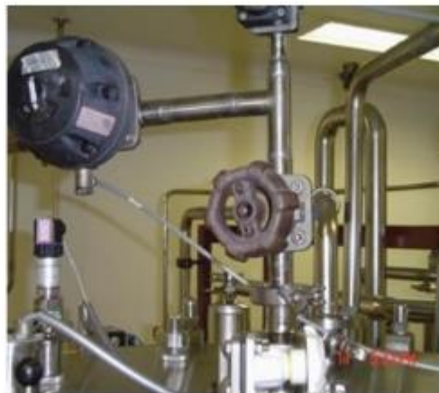
Mechanical modification for spray ball connection to perform CIP
